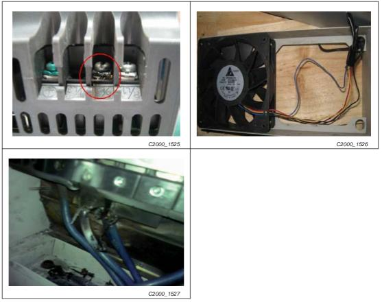
Fig. 18-5: Poor wiring is an often error cause
